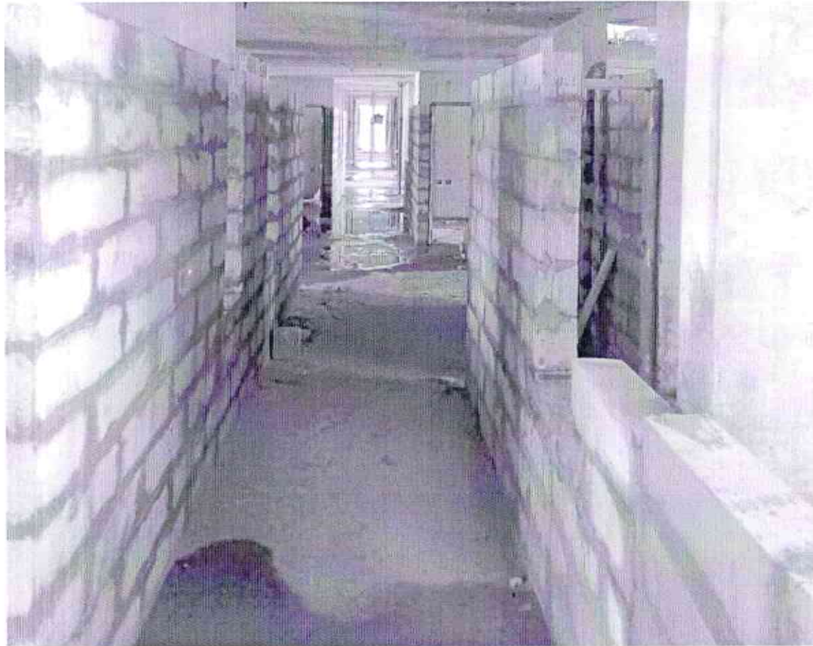
C Block Corridor
