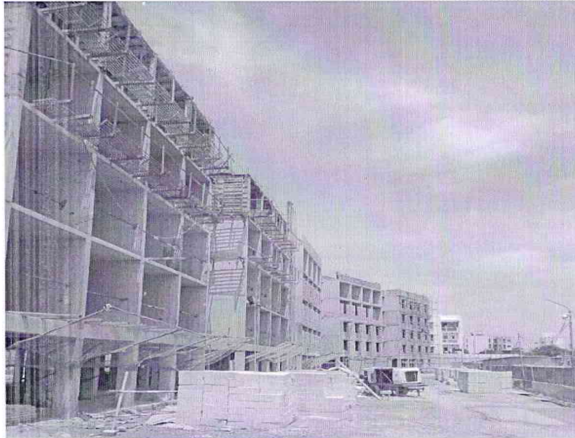
C Block External North Side
