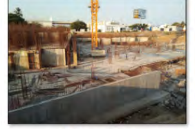
Raft Concrete work
