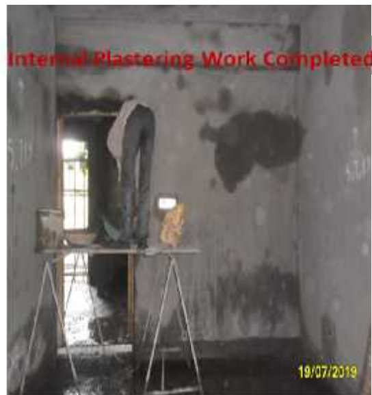
Internal Plastering Work Completed
