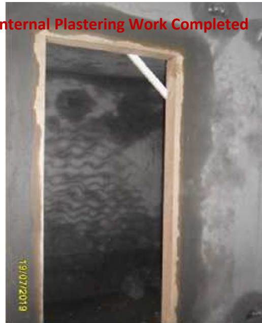
Internal Plastering Work Completed
