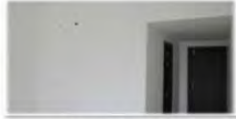
Door finishing works
