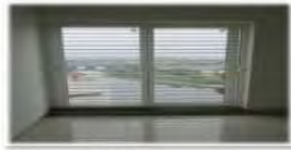
UPVC & Grill fixing works
