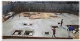
STP roof completed
