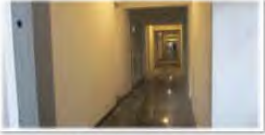
Corridor flooring works
