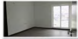
Wooden flooring & Grill fixing works
