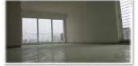
Flooring & Painting works
