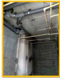
Water proofing & Plumbing works
