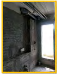
Water proofing & Plumbing works 3
