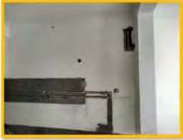
Water proofing & Plumbing works 2
