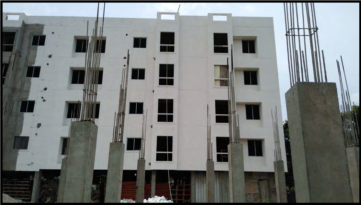
WEST ELEVATION OF BUILDING
